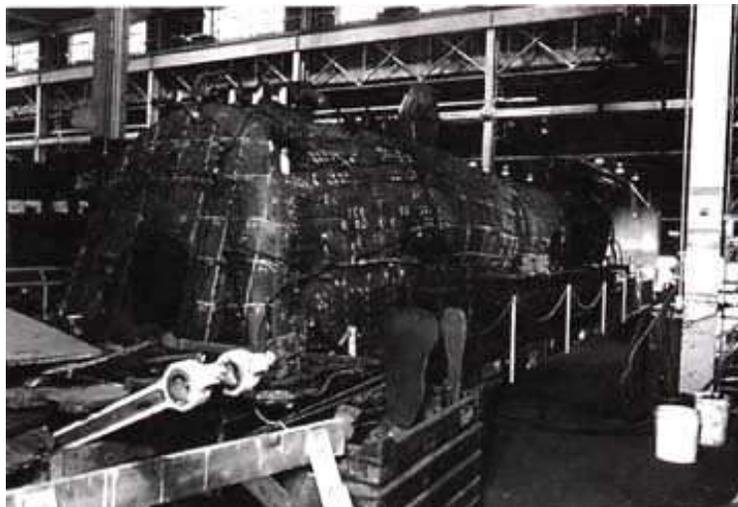
**Overall view of engineer's side of B&M 3713 showing cab removed with staybolts visible.**
